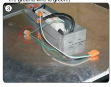
Cut off the electricity, insert the L, N and Ground wires of junction box on the ceiling into terminal B. (Note: Ground wire should be in the middle socket of the terminal.)
