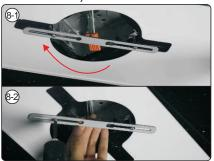
Pull down the terminal B of junction box on the ceiling, connect it to terminal A of LED Panel Light.
