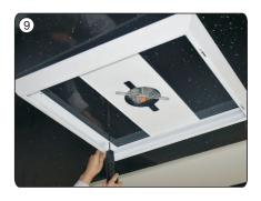
Mount the kit when the kit groove and connect plate are aligned, rotate the kit to your preferred position, then tighten the two screws on the junction box.
