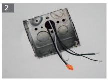
**Step 2:** Turn off power. Insert the L, N wires of the J-Box into the male connector.
