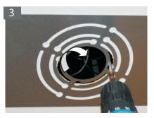
**Step 3:** Align the holes on the surface mounted kit with the holes on the J-Box. Tighten 2 #8-32 screws, rotate the plate to your desired position and fasten the KA3.5x20mm screws into the ceiling until the kit is flush with the ceiling.
