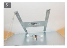
**Step 5:** Attach the metal cable on the hook.
