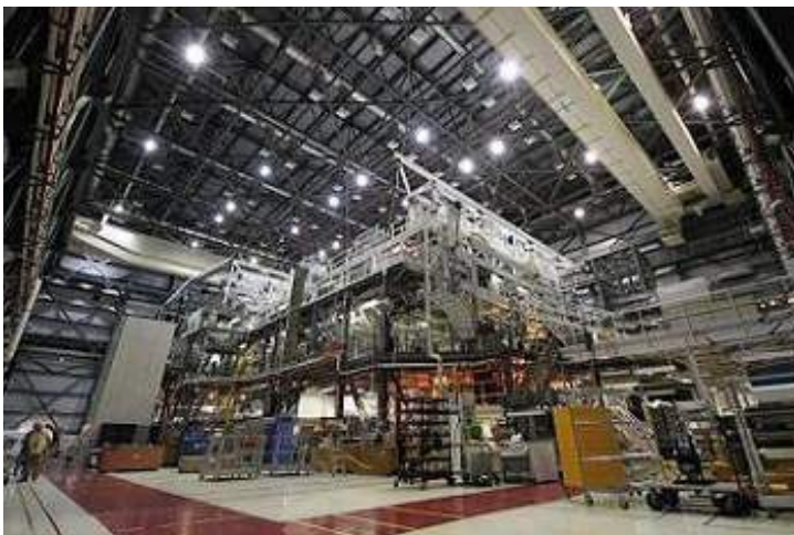
BEFORE: 1000W HPS High Bays
