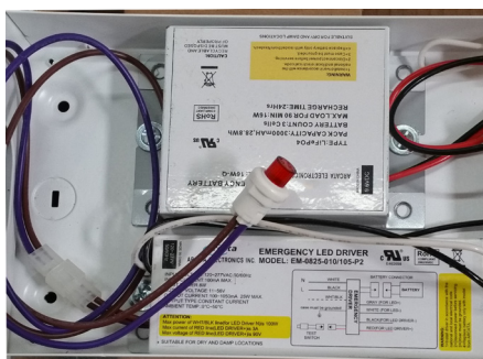
Emergency Battery Backup Driver
